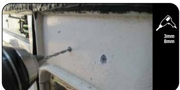
Drill 3mm pilot holes and then open each hole with an 8mm drill bit.
